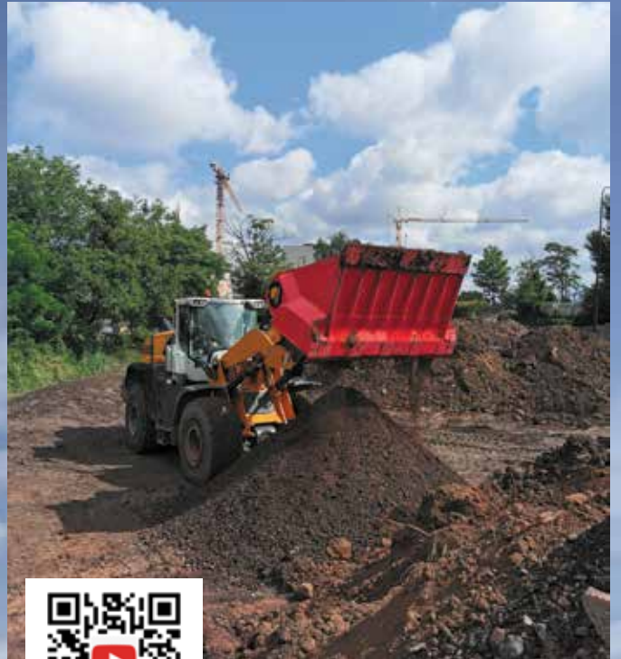
TOPSOIL SCREENING
